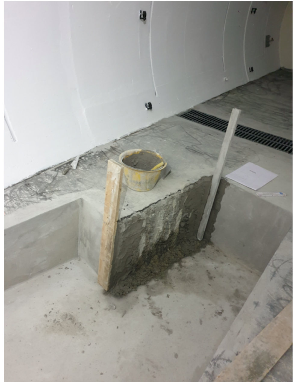
Extending the trench for FASERv
